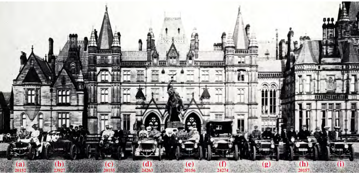
The Motor Union meeting at Eaton Hall, Cheshire, July 15, 1905, with three of the five production Rolls-Royce models represented: 10 hp 2-cyl. (a, c, e, and h), 20 hp 4-cyl. (d), 30 hp 6-cyl. (b and f), and two of the three Royce prototypes (g and i). Note the different radiator designs of the nearly identical Royce prototypes and the Rolls-Royce between them.
